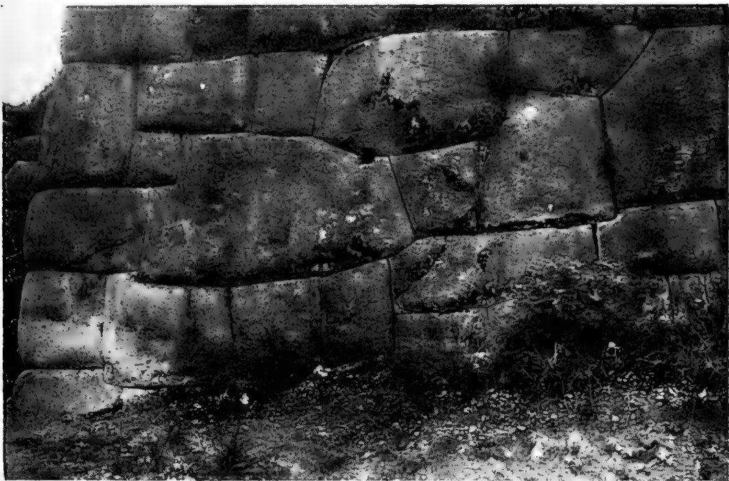
FIG. 72.—A portion of a wall in the great Inca fortress near Cuzco. The stones are fitted with great exactness, but without mortar. A drainage opening is shown in center. The corner stones are rounded and the wall slopes a little. The Incas had no beasts of burden (the llama will carry 75 pounds, but will not pull in harness) and no metal tools. Some of the large stones weigh many tons.
